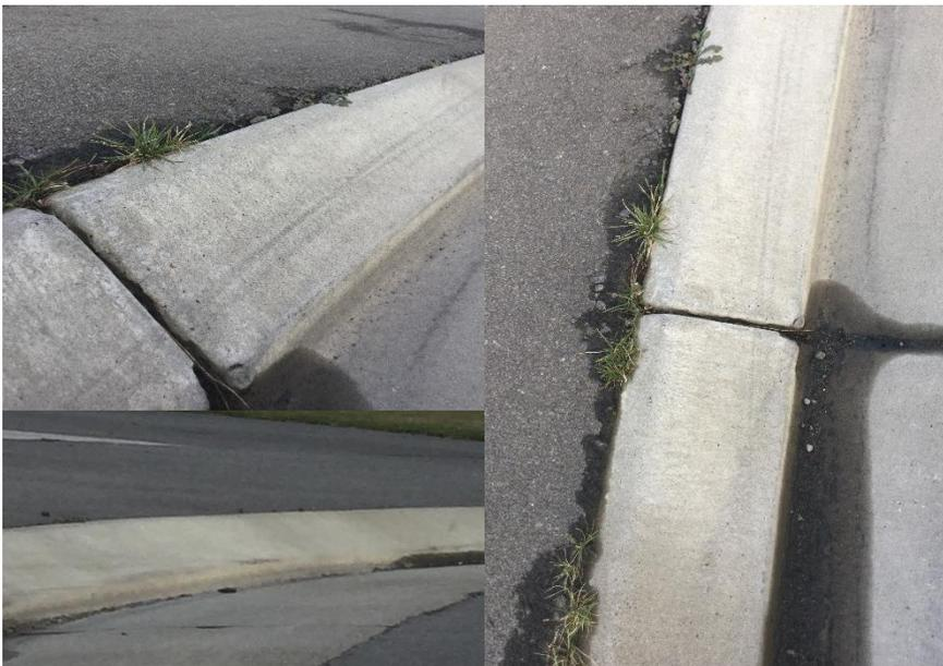
**Figure 3: Low profile kerb and channel design**
