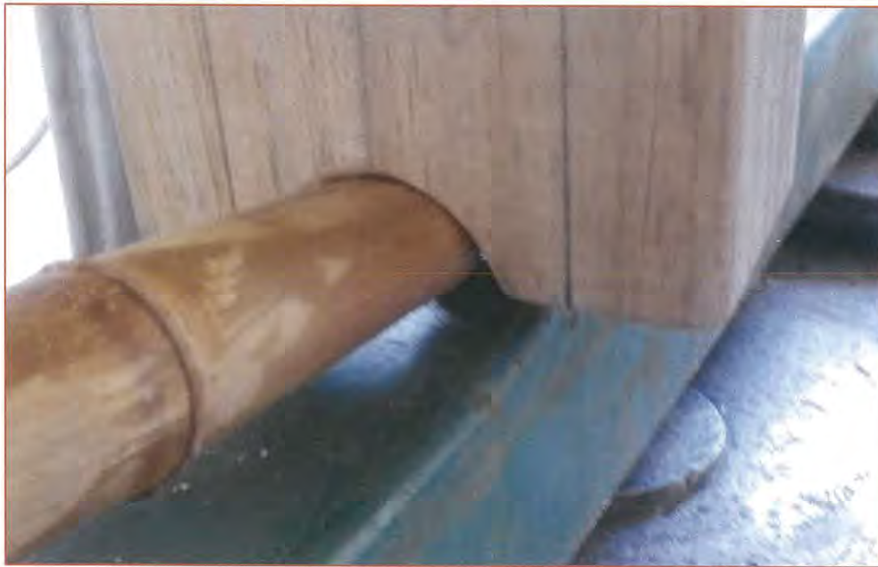
Figure 7-6: Crush failure at edge of support possibly due to insufficient ability for support to rotate.
