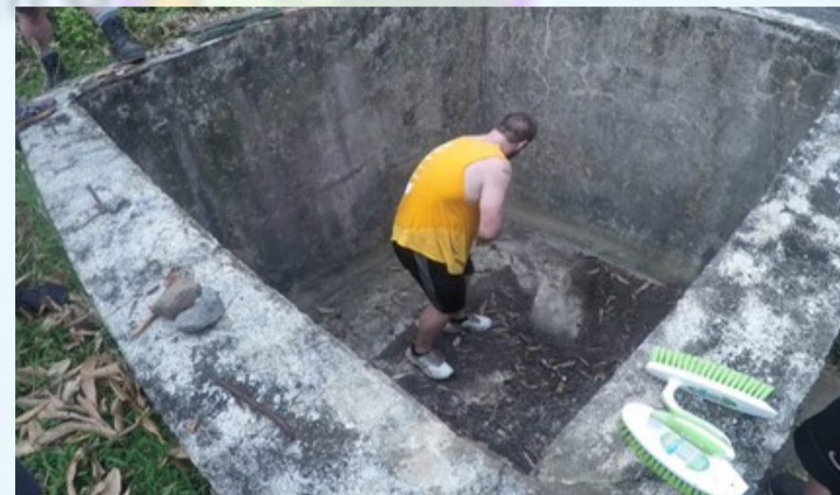
Figure 2: Tank cleaned out
